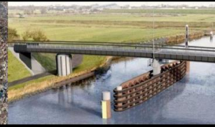
Bicycle bridge from bio-based composite materials, e.g. timber, resin, etc. (Leeuwarden/NL)
