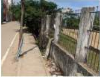
North Side Compound Wall
