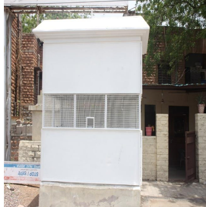
Police cabin after paint
