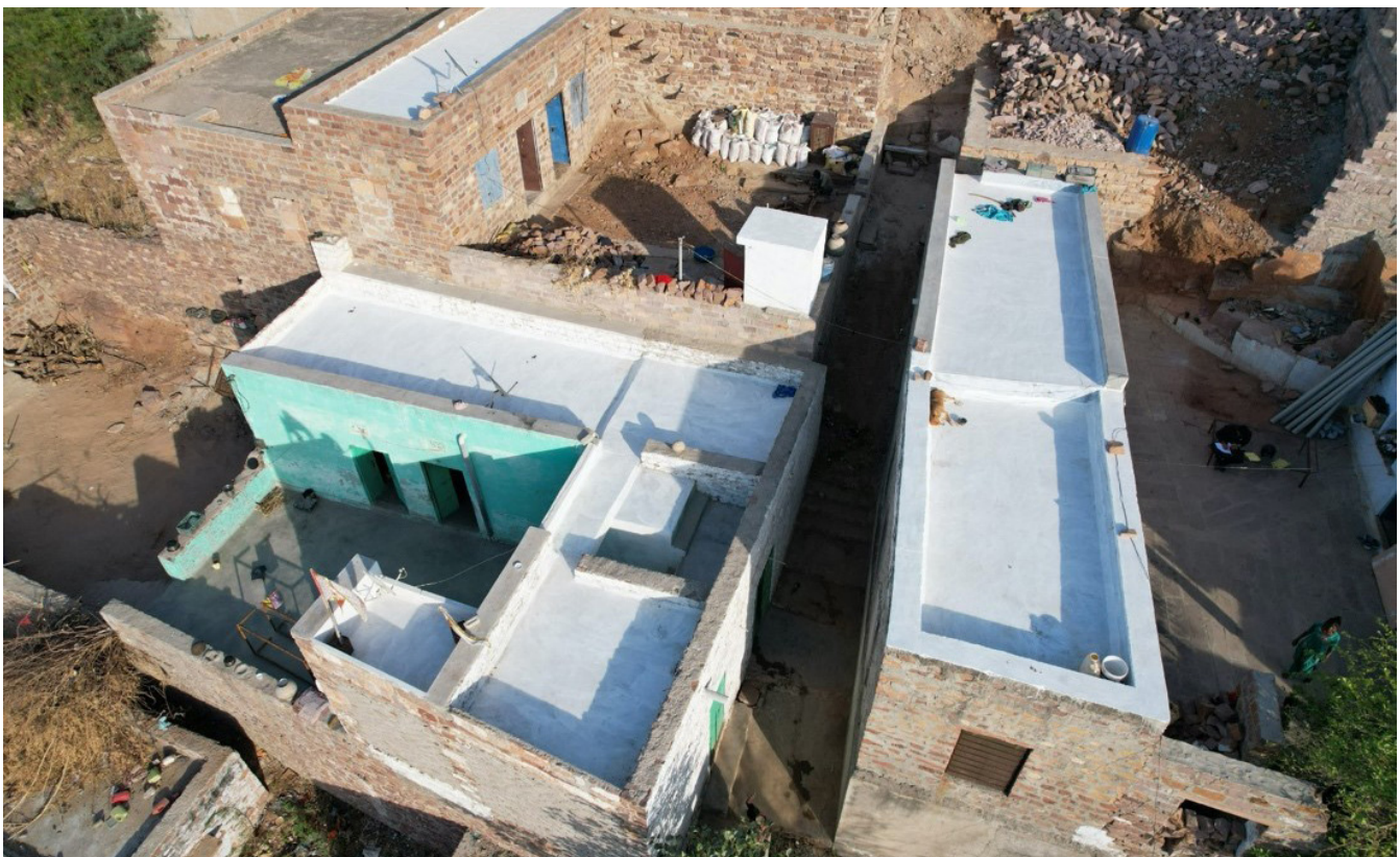
Figure 18: Houses with cool roof paints deployed to adapt to extreme heat in Jodhpur, India (Credit: Mahila Housing Trust)
