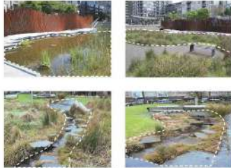
Fig. 2.23 Includes permeable paving, vegetative and biofiltration basins
