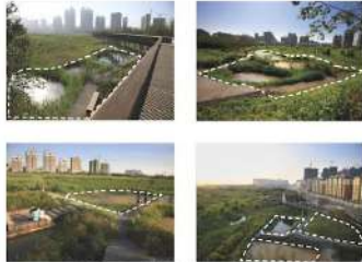
Fig. 2.32. Integrals vegetated swales that capture and filter stormwater.
