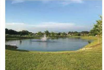
Fig. 2.55 Reference - Retention Pond
