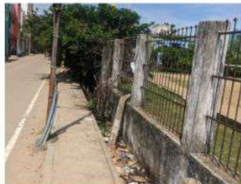
North Side Compound Wall
