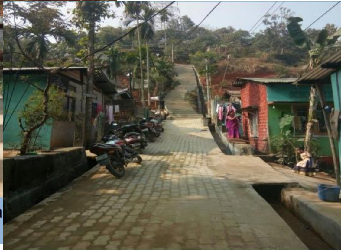
Roads with paver blocks and drain with step chutes
