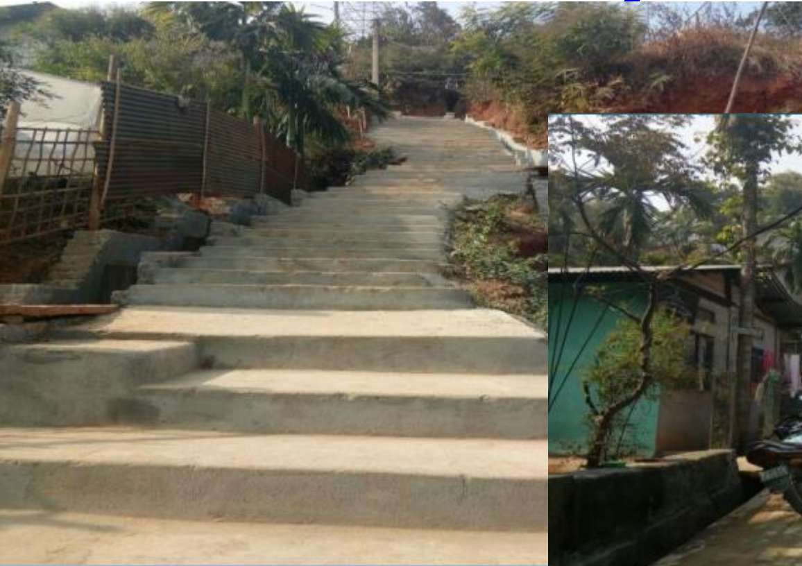
Old road repaired and New Dra step chutes
