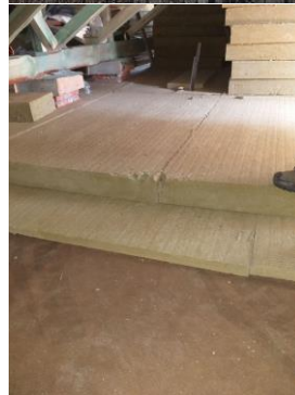
Insulation Of top floor ceiling
