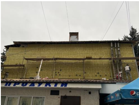
View from North
