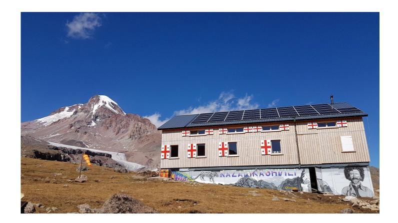
15 KW off Grid PV Plant– Powering ALTIHUT (3014M a.s.) and also the GSM network system, to ensure the stabile communication for the tourists in the tourist's area.
