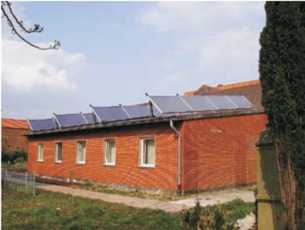
Solar panels on roofs are a part of the vision for a sustainable settlement
