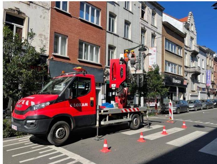
Installation with Loxam
