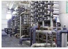
Seawater desalination plant in Ghana Basic engineering of a: reverse osmosis, ultrafiltration and re-mineralization plant with a 60,000 m³- day capacity that will supply different towns near Accra
